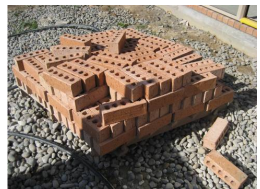
Bricks returned to supplier for reuse © Copyright
