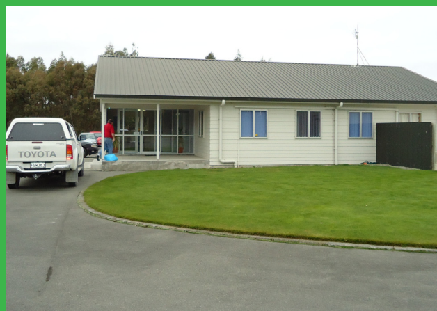
MRP administration building © Copyright
