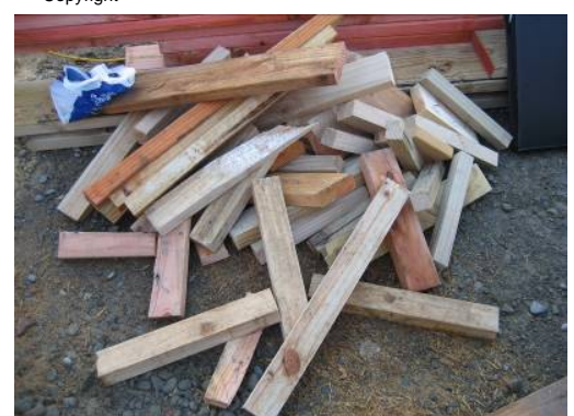
Timber off-cuts in separate piles for reuse © Copyright
