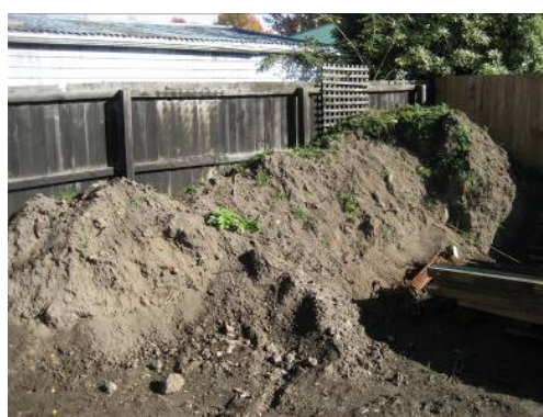
Soil stockpiled for reuse on-site © Copyright
