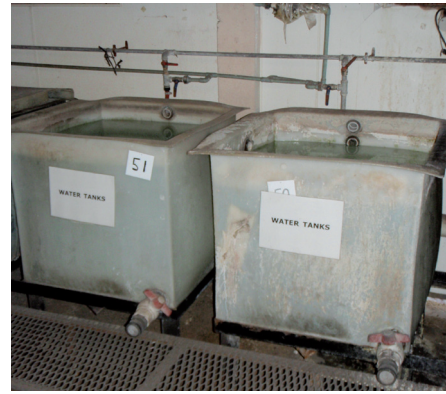
Cleaning basin water reuse system © Copyright
