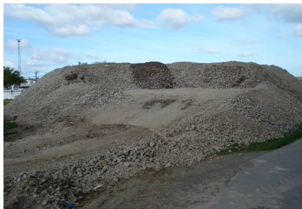
Concrete crushed for reuse on-site © Copyright
