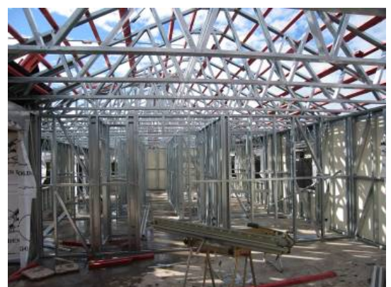
Steel framing © Copyright
