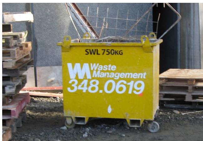
Bucket skips used to transport waste to the central sorting area © Copyright
